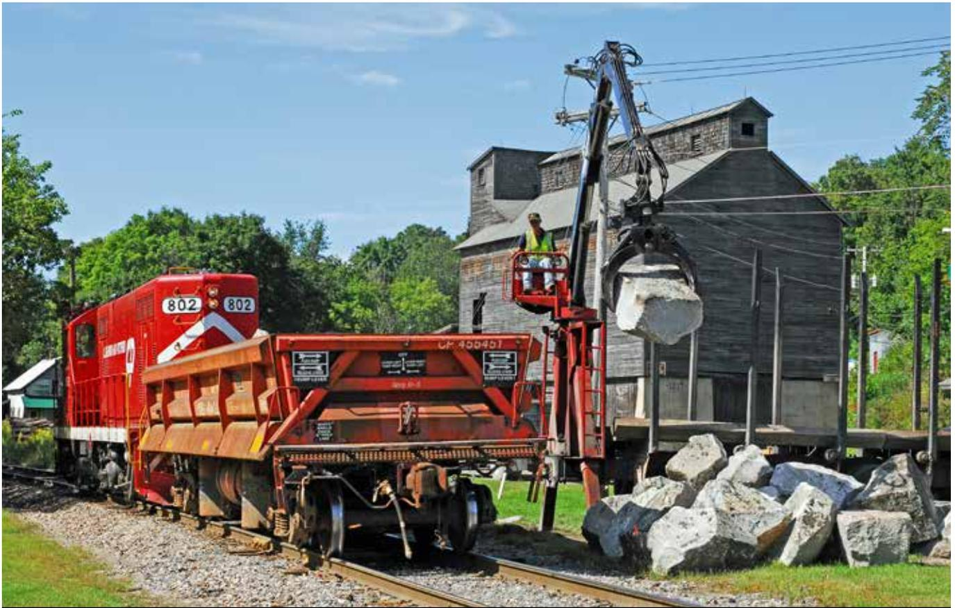
**As part of repairs in the aftermath of Hurricane Irene, which shut down some lines for three weeks, a Vermont Rail System train takes on rocks in Brandon, Vt., for repair of a storm-damaged embankment along the right-of-way in September 2011.** Kevin Burkholder
